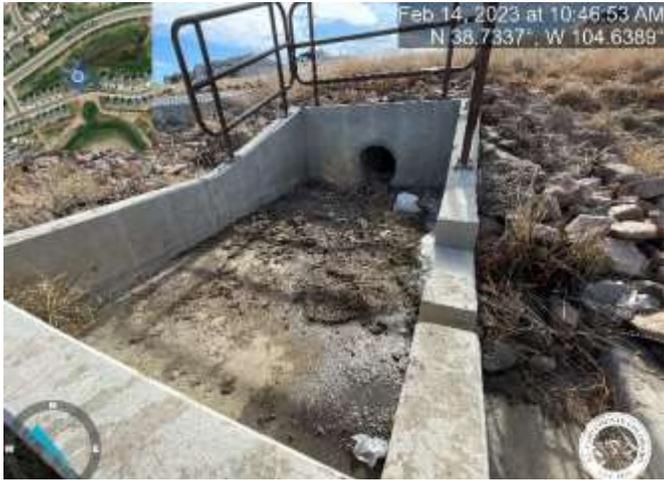
Photo 5: Forebay No. 2A: Clean sediment and debris out of forebay and pipe.
