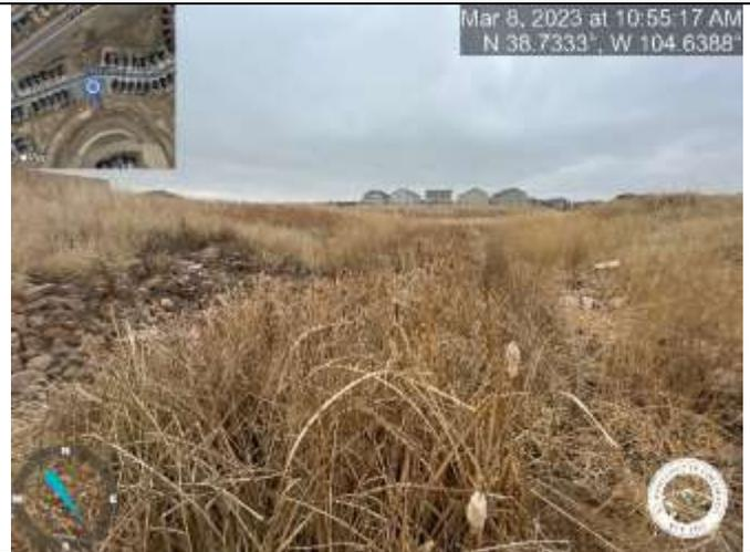
Photo 26: Pond C1-R: Note that this is not an FA item, but a maintenance item, just listed here as an FYI: Advise cleaning out the outfall area and create positive drainage.
