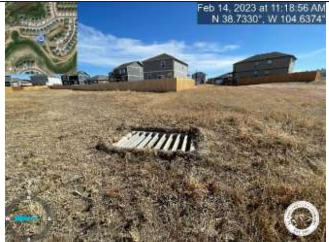
Photo 10: Tract F Inlet DP-12: Remove temporary control measure straw wattle.
