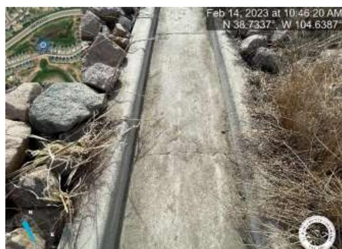
Photo 3: Forebay No. 2B: Repair crack in trickle channel.
