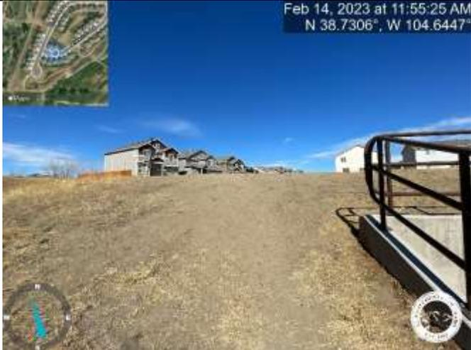
Photo 19: Pond CR2: Failure to achieve uniform vegetative cover with an individual plant density of at least 70 percent along slope along the north slope.
