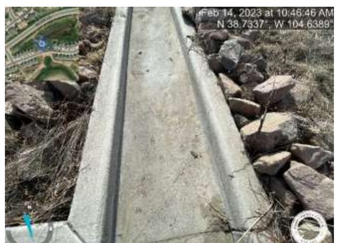
Photo 4: Forebay No. 2A: Repair crack in trickle channel.
