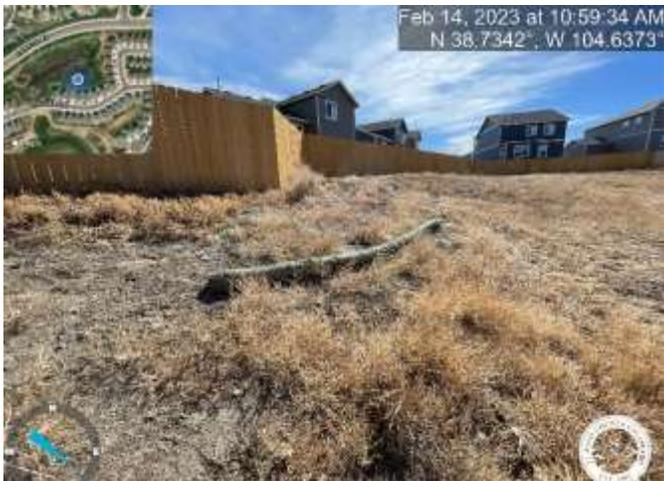
Photo 7: Behind Forebay No. 1: Remove old roll of Erosion Control Blanket.
