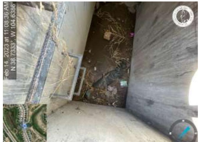
Photo 8: Inlet DP-10: Remove sediment and debris from inlet (inlet is marked with a green dot on the lid).
