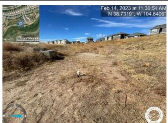
Photo 12: Pond CR3: Remove vegetation from the base of the sand filter basin.
