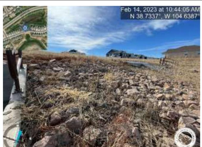
Photo 2: forebay No. 2B: Failure to implement soil rip rap per approved plans. Page C9.8 Creekside at Lorson Ranch filing No. 1 Street and Storm Sewer Construction Plans.
