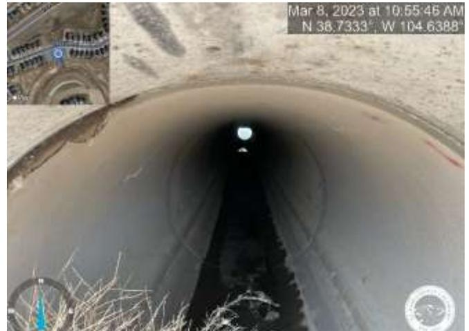
Photo 24: Pond C1-R: Note that this is not an FA item, but a maintenance item, just listed here as an FYI: Advise cleaning out the outfall area and create positive drainage.
