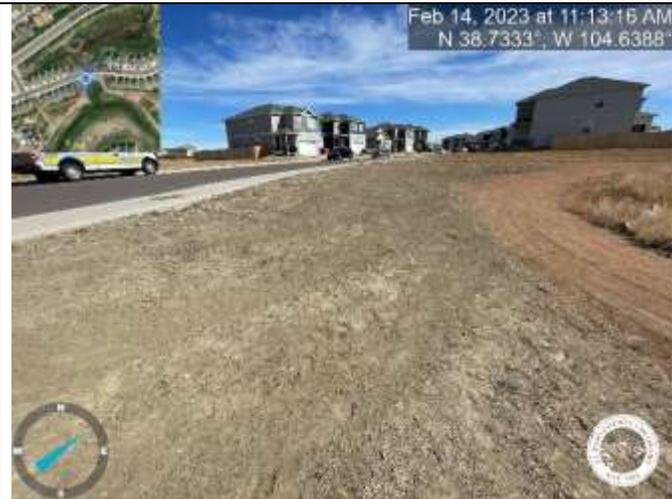
Photo 9: STA 22+65.10: Failure to achieve uniform vegetative cover with an individual plant density of at least 70 percent along slope.
