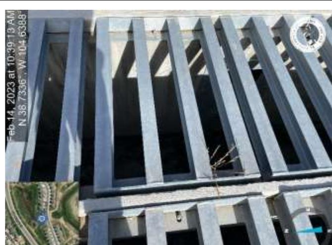
Photo 1: Pond C1-R: Implement missing bolts on outlet structure top grates (approximately 11 missing).
