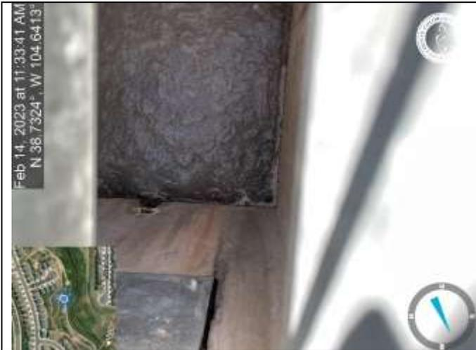
Photo 13: Pond CR3: Failure to implement Steel Restrictor Plate. Reference page C9.4 Creekside at Lorson Ranch filing No. 1 Street and Storm Sewer Construction Plans.
