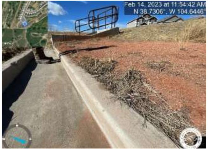
Photo 18: Pond CR2: Remove sediment to match the top of trickle channel curb with a 3% slope towards trickle channel for positive drainage.
