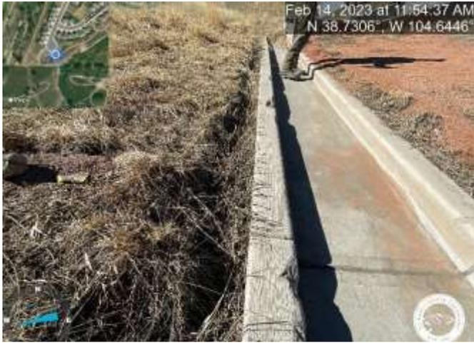
Photo 17: Pond CR2: Raise pond bottom to top of trickle channel curb with a 3% slope towards trickle channel for positive drainage.
