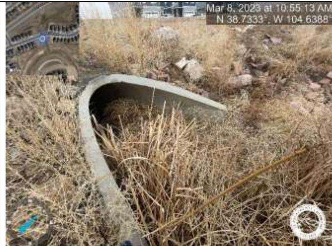
Photo 25: Pond C1-R: Note that this is not an FA item, but a maintenance item, just listed here as an FYI: Advise cleaning out the outfall area and create positive drainage.
