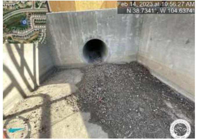
Photo 6: Forebay No. 1: Clean sediment and debris out of forebay and pipe.
