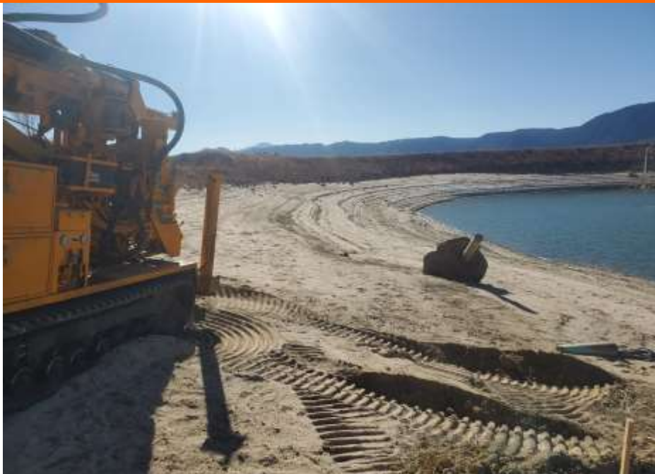
Near Boring SB-1 Facing Southwest
