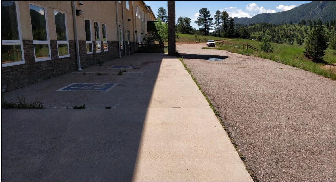
Photograph 3. PCC/AC Apron Southwest of Existing Building - Looking Southeast
