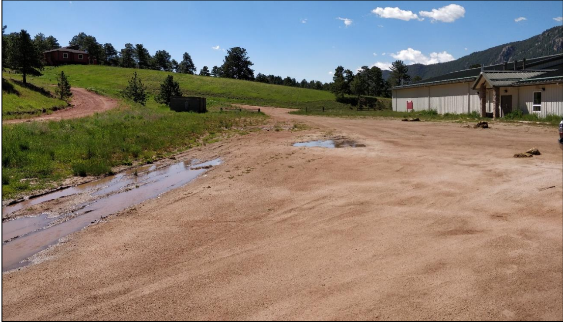
Photograph 1. Parking Lot North of Building - Looking Southeast
