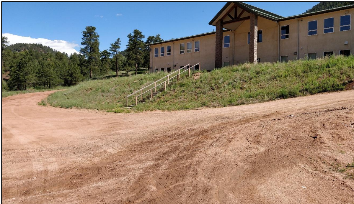
Photograph 4. View of Southwest Side of Existing Building – Looking North
