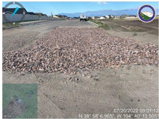
VTC has been lengthened and scarified.
