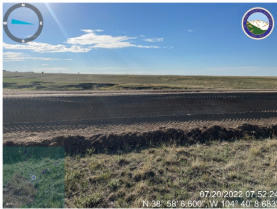
Compact Berm implemented around perimeter of Homestead North.
