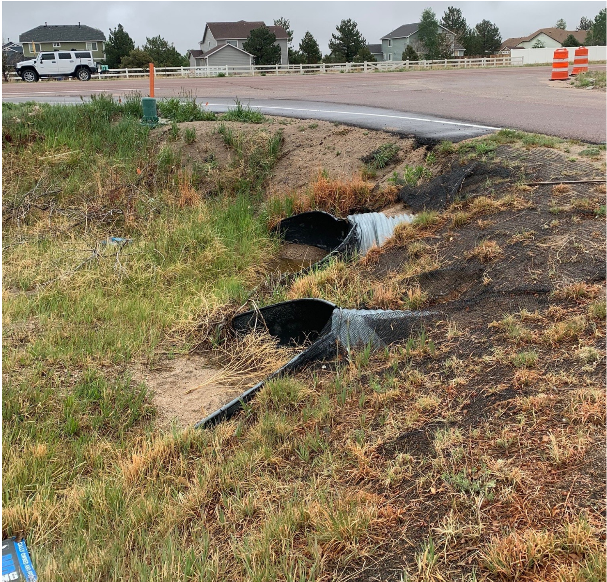
Existing 2-36" CMP under Owl Place (Upstream Inlets)
