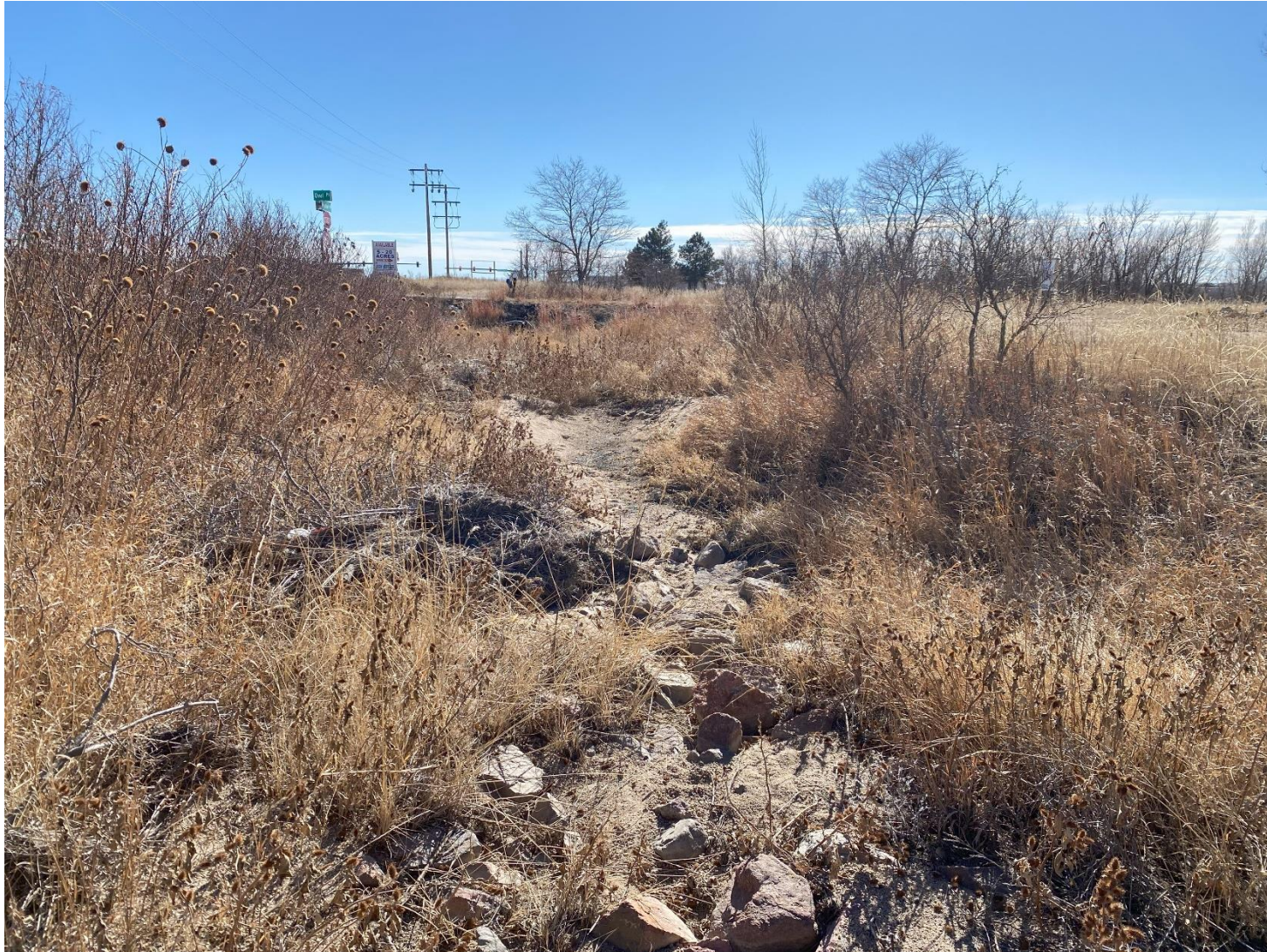
Photo 2 – Another view facing south of the constructed ditch and OHWM, just north of OHWM SP1. The confluence between the ditch and W1 can be seen in the top half of the photo. Rock riprap has been installed in this section of the ditch and can be seen in the photo.
