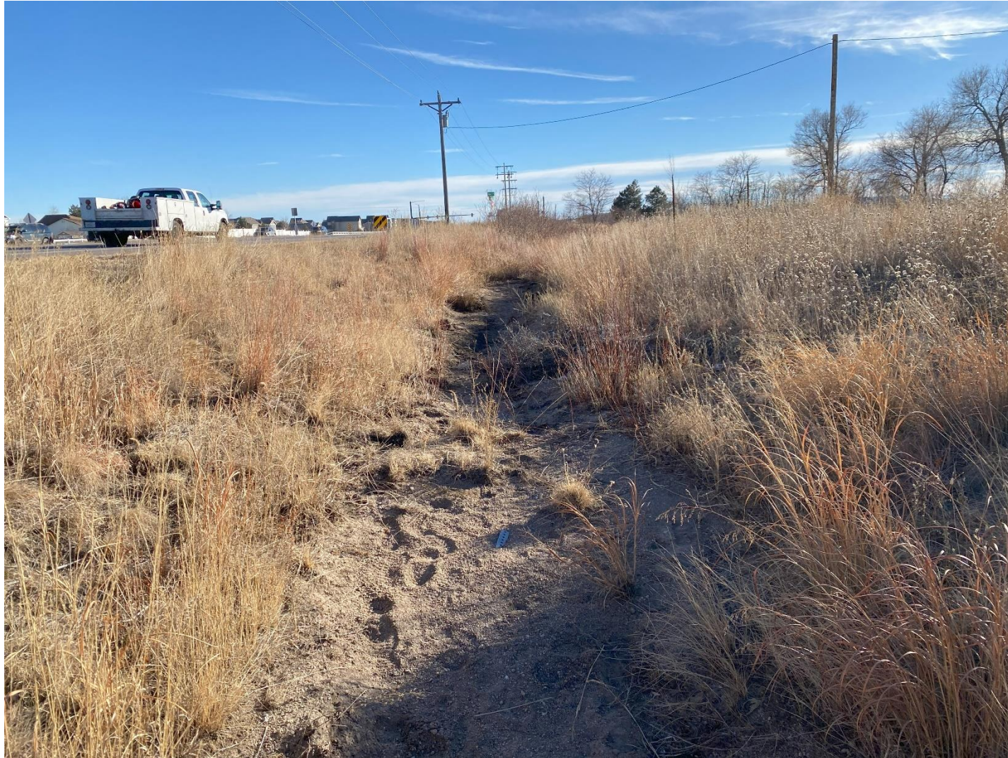
Photo 1 – View facing south of the constructed ditch showing the topographic, sediment, and vegetation changes of an OHWM; the ditch eventually connects with Wetland 1 to the south.
