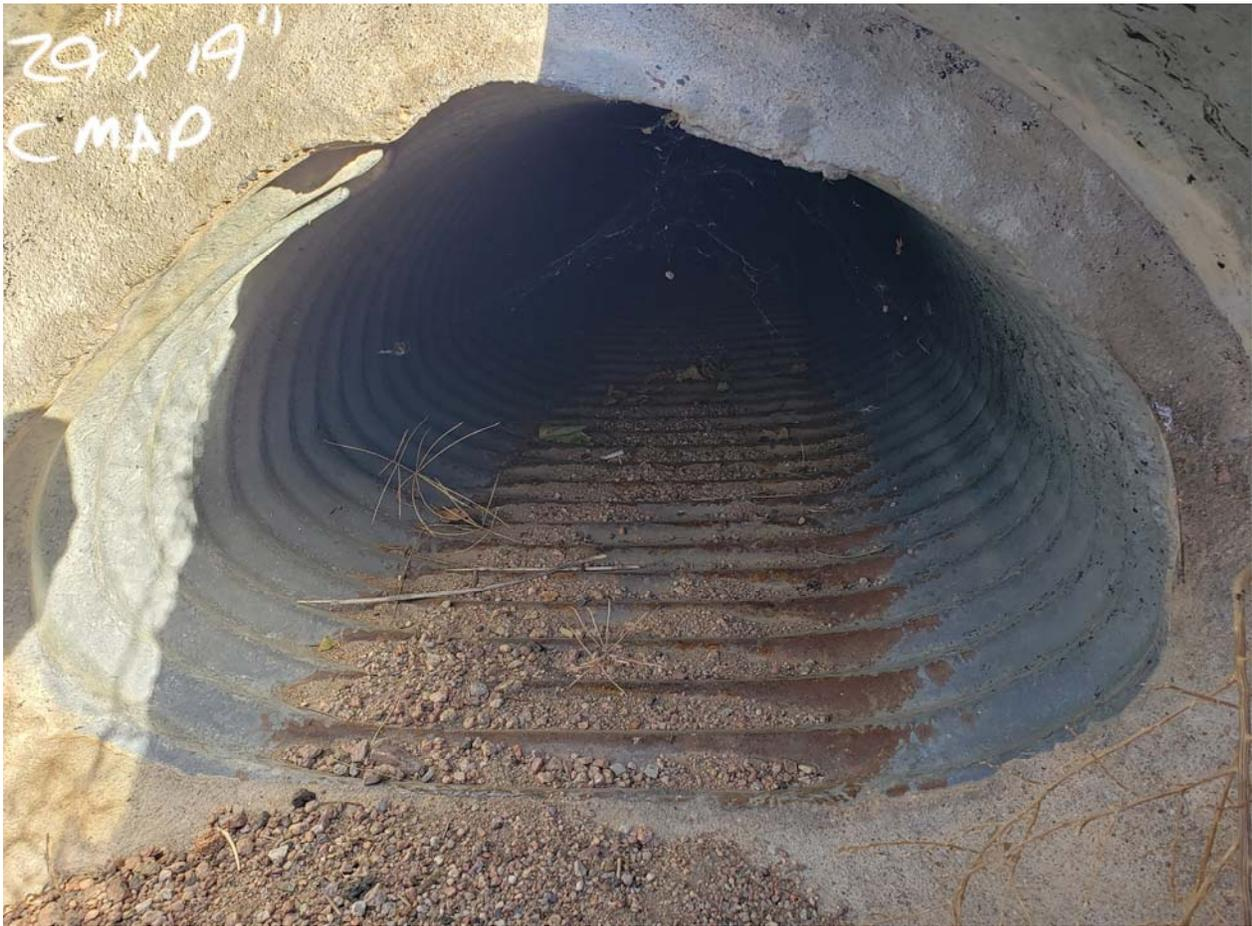
*Figure 5-Existing 29" x 19" CMAP Fontaine Road Ditch Across Rolling View Drive (Appears to be grouted in insert)
