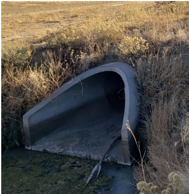
*Figure 6-Existing 60" RCP FMIC Culvert in Glens at Widefield Filing No. 6 (South of Corvallis)*
