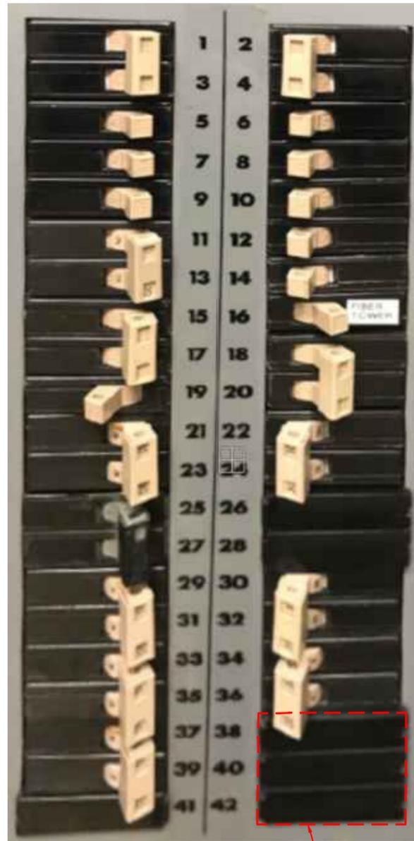
(3) PROPOSED 20 AMP BREAKERS FOR BLOCK HEATER, BATTERY HEATER, AND BATTERY CHARGER ON NEW AT&T GENERATOR
