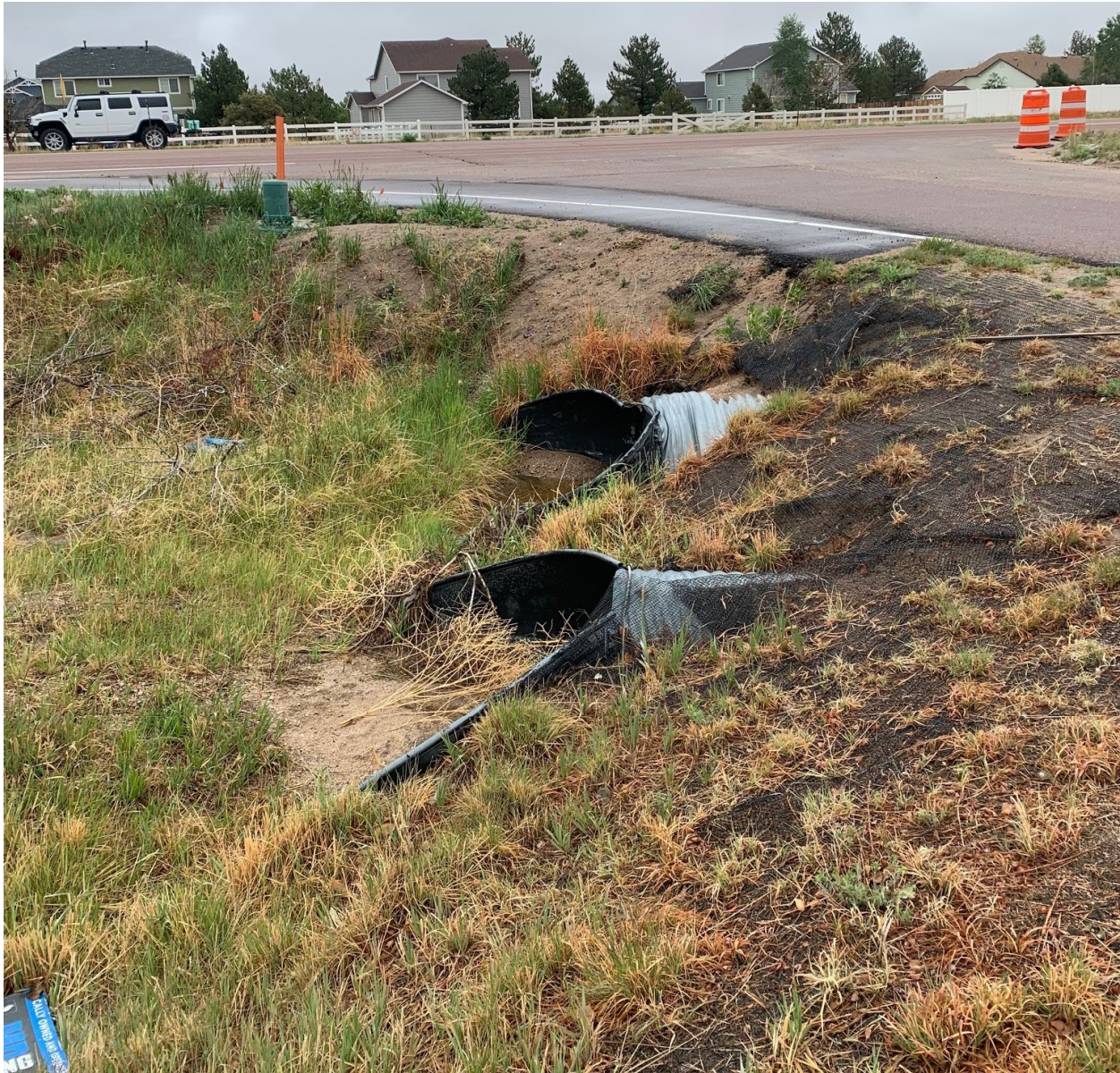
Existing 2-36" CMP under Owl Place (Upstream Inlets)
