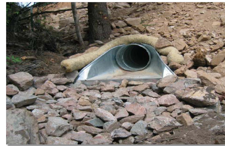
Photograph TOP-1. Riprap outlet protection.
