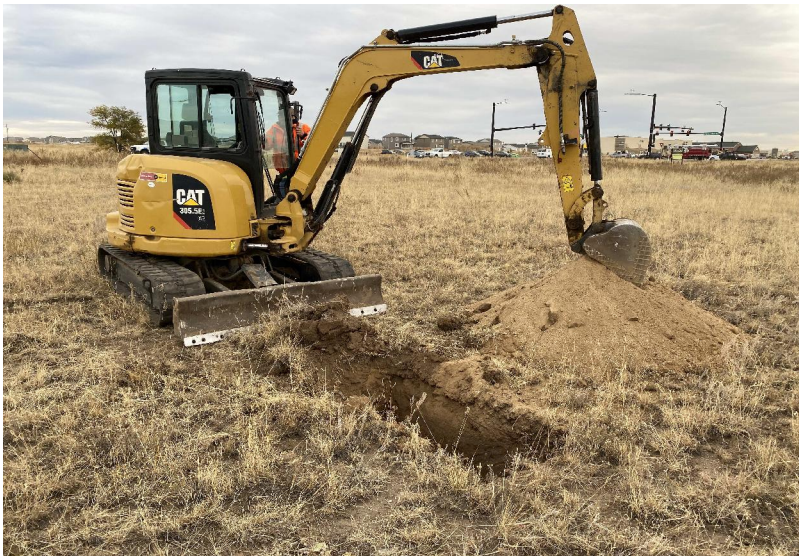
3. Overall view of excavation for Test Pit 1
