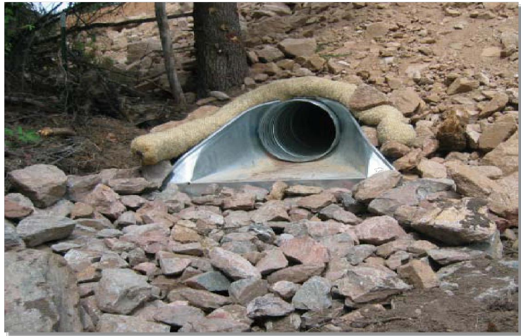
Photograph TOP-1. Riprap outlet protection.
