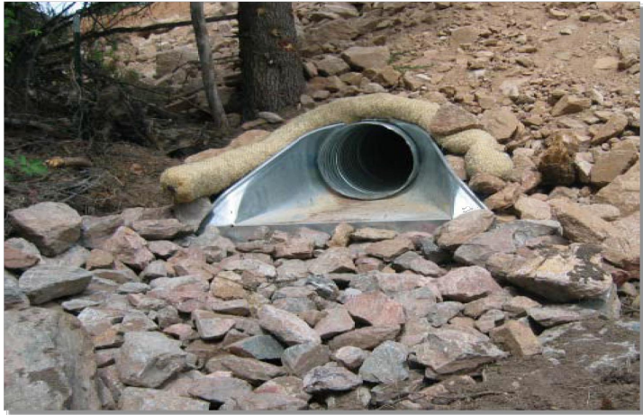
Photograph TOP-1. Riprap outlet protection.
