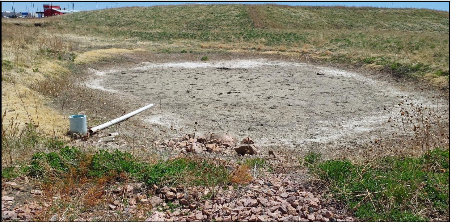
Photo No: 9 Direction Photo Taken: Southeast Figure No: 4 Description: Overview of Wetland C, located in a dry sediment basin. A cobble riprap drainage swale in the foreground.
