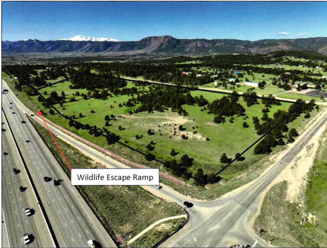
Photo 1. Looking SW at the project site.
