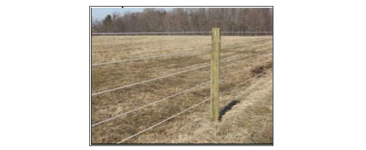
G SMOOTH WIRE RANCH FENCE (6'-7' HEIGHT) NOT TO SCALE
