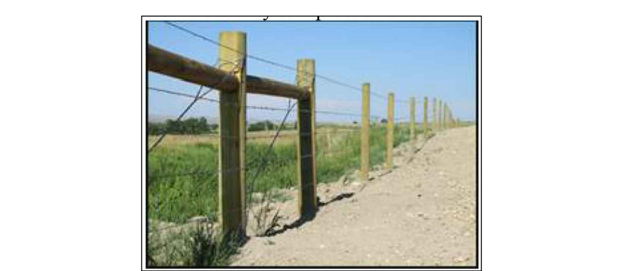
H BARBED WIRE FENCE NOT TO SCALE
