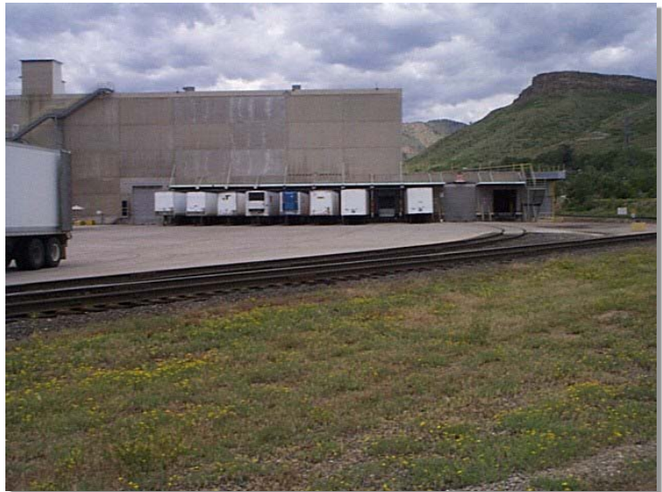
Photograph CS-1. Covered truck loading dock helps reduce exposure of materials to runoff.
