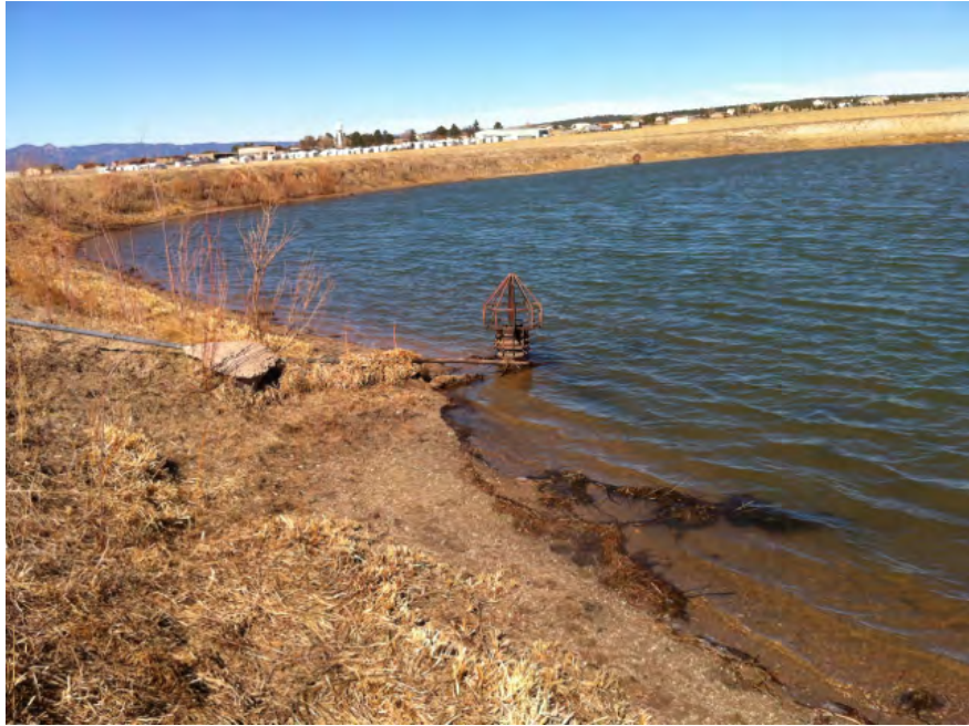
Pond 4 – Looking northwest from dam. This deep pond has a sparse, narrow wetland fringe. The pond drains via the standpipe, to a culvert under the dam, and into Pond 5. Pond 5 is a small open water area (~6' diameter). 3/16/15
