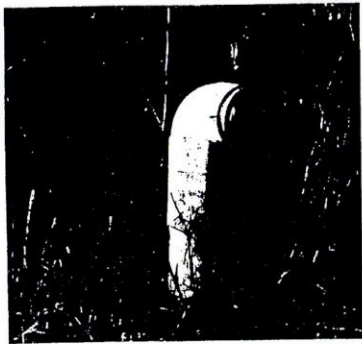
Figure B-5-1(a) Dry hydrant.
