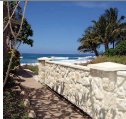
▲ Lava Rock Privacy Wall
