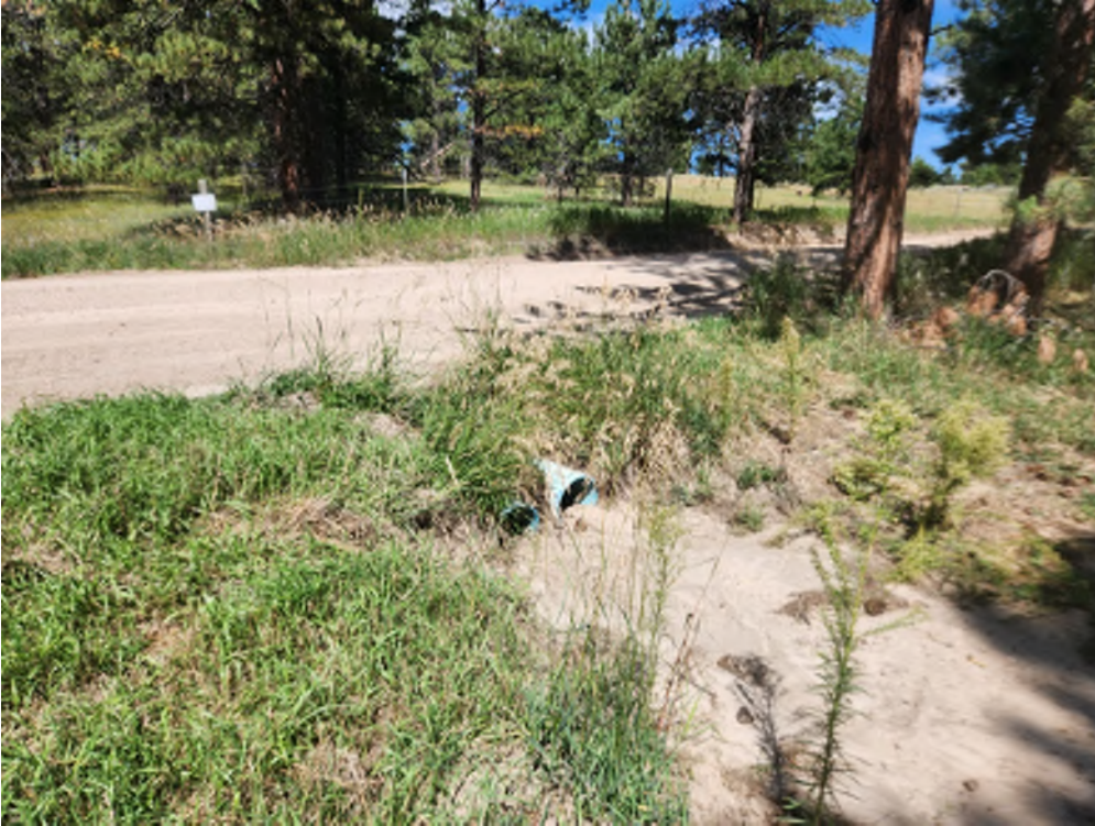
Figure 8: Double 12" PVC culverts, headwater
