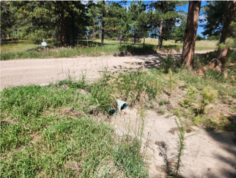
Figure 8: Double 12" PVC culverts, upstream
