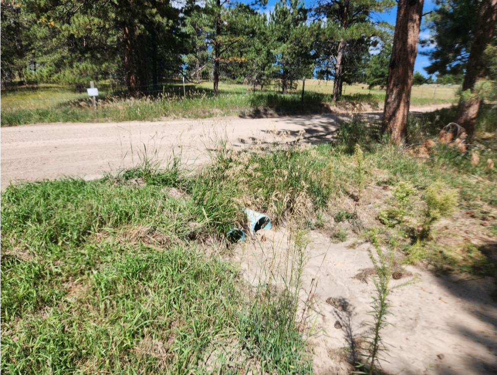
Figure 8: Double 12" PVC culverts, upstream
