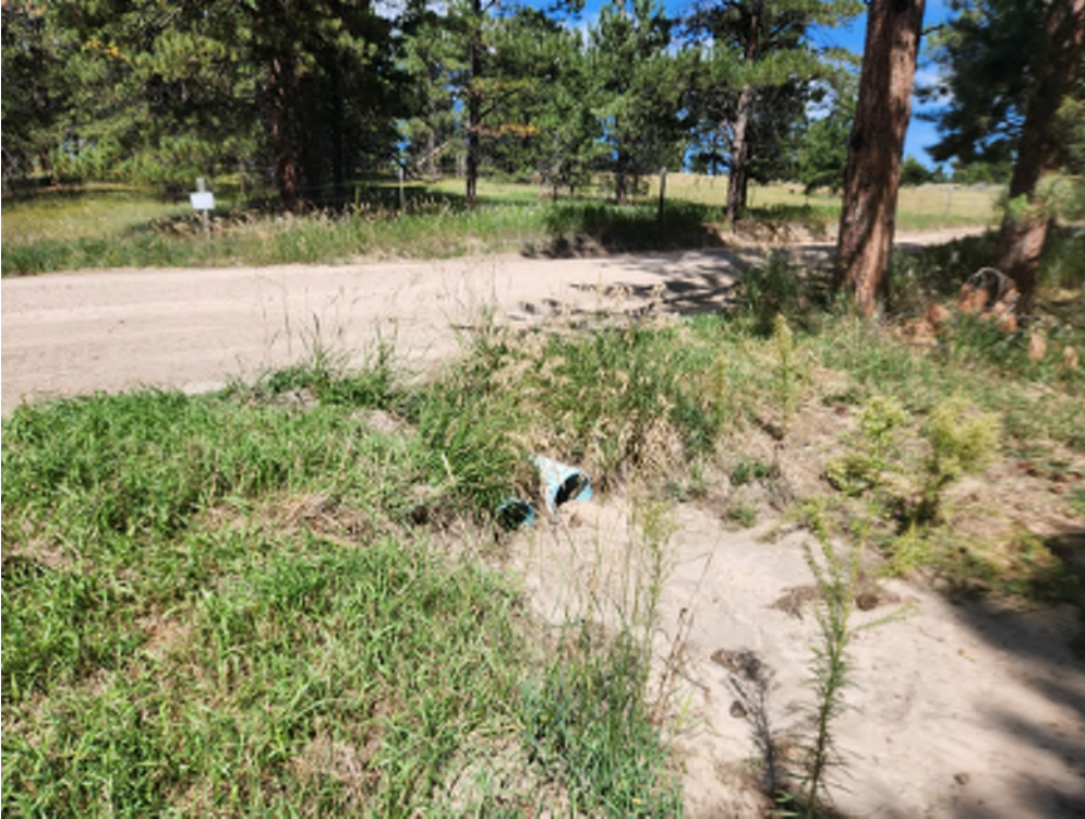
Figure 8: Double 12" PVC culverts, headwater
