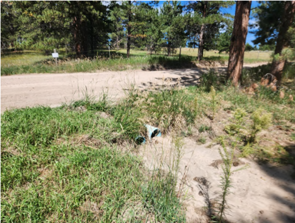
Figure 8: Double 12” PVC culverts, headwater
