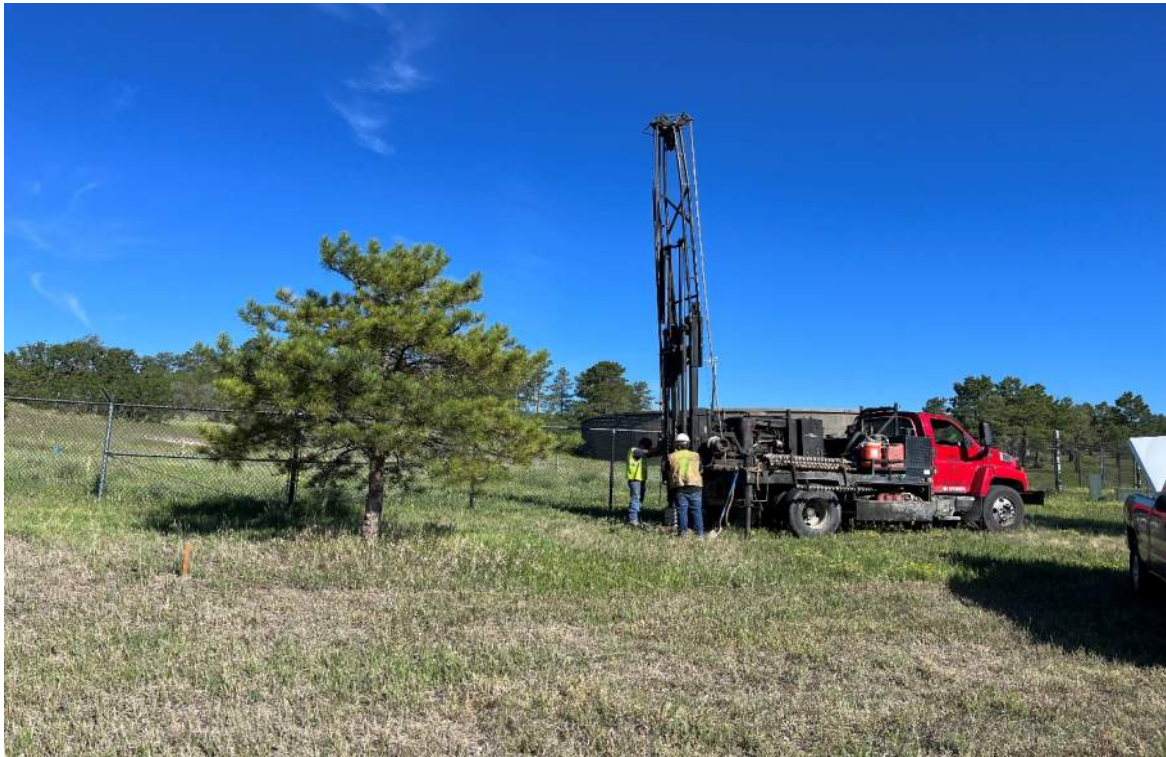
DRILLING BORING BH-1 - LOOKING NORTHWEST
