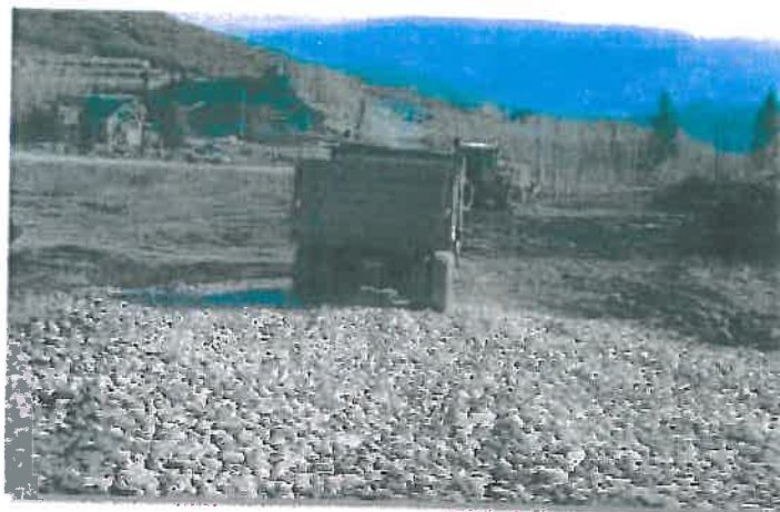
Photograph VTC-1. A vehicle tracking control pad constructed with properly sized rock reduces off-site sediment tracking.
