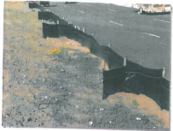
Photograph SF-2. When silt fence is not installed along the contour, a "J-hook" installation may be appropriate to ensure that the BMP does not create concentrated flow parallel to the silt fence. Photo courtesy of Tom Gore.
