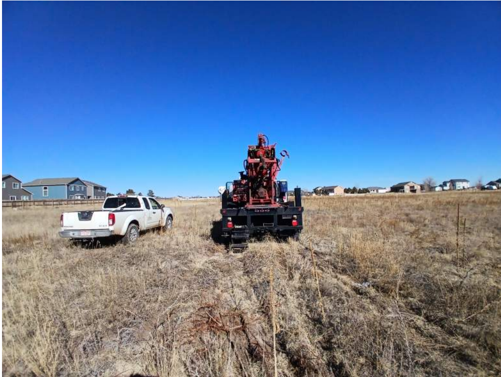
SITE CONDITIONS AND DRILLING AT BORING B-6 - LOOKING NORTH
