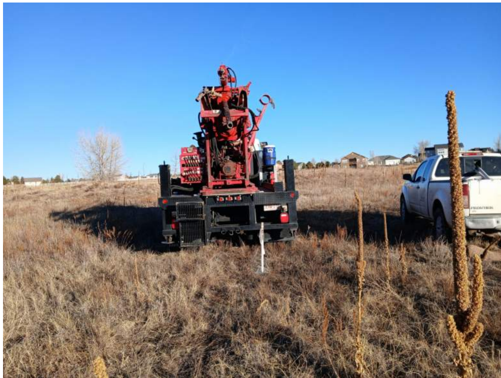
SITE CONDITIONS AND DRILLING AT BORING B-9 - LOOKING EAST
