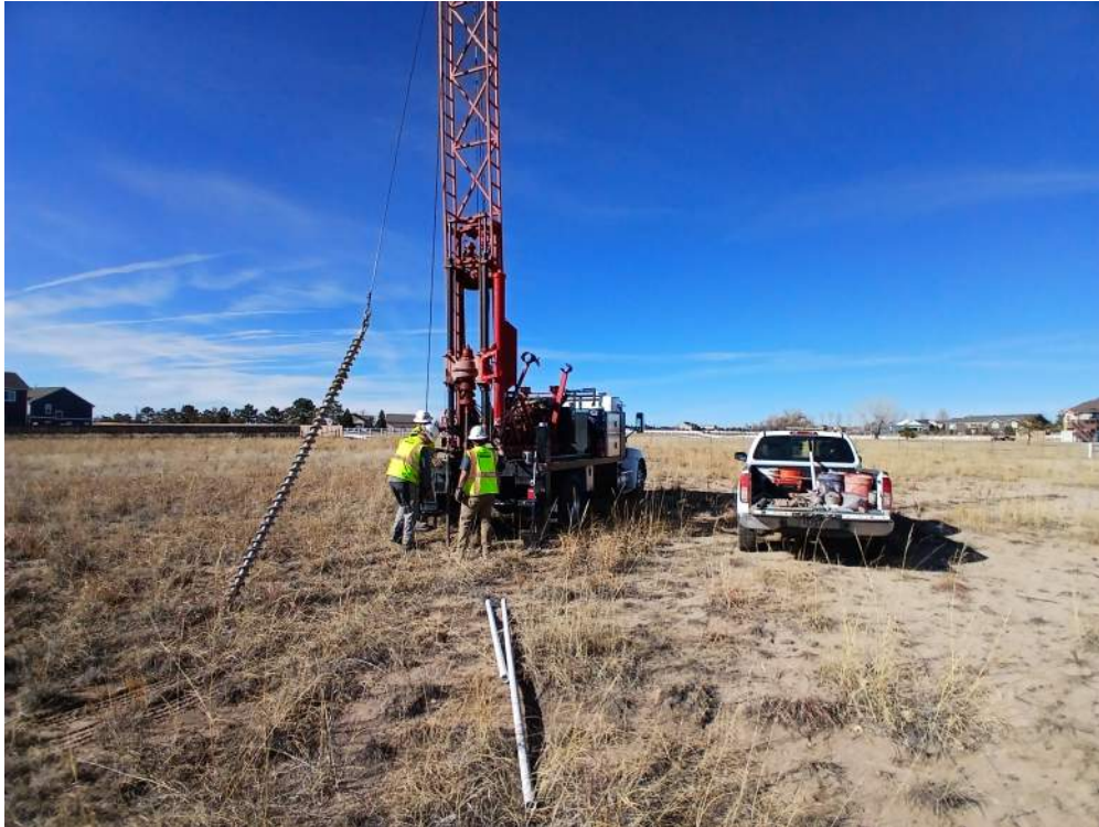
SITE CONDITIONS AND DRILLING AT BORING B-2 - LOOKING NORTH
