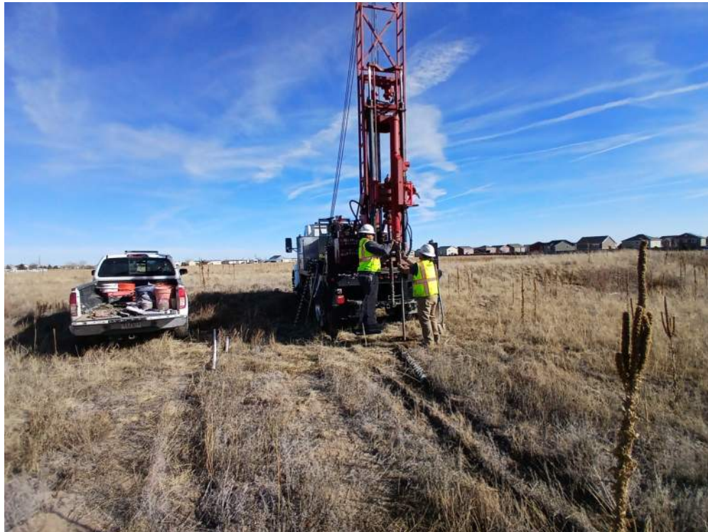
SITE CONDITIONS AND DRILLING AT BORING B-3 - LOOKING EAST
