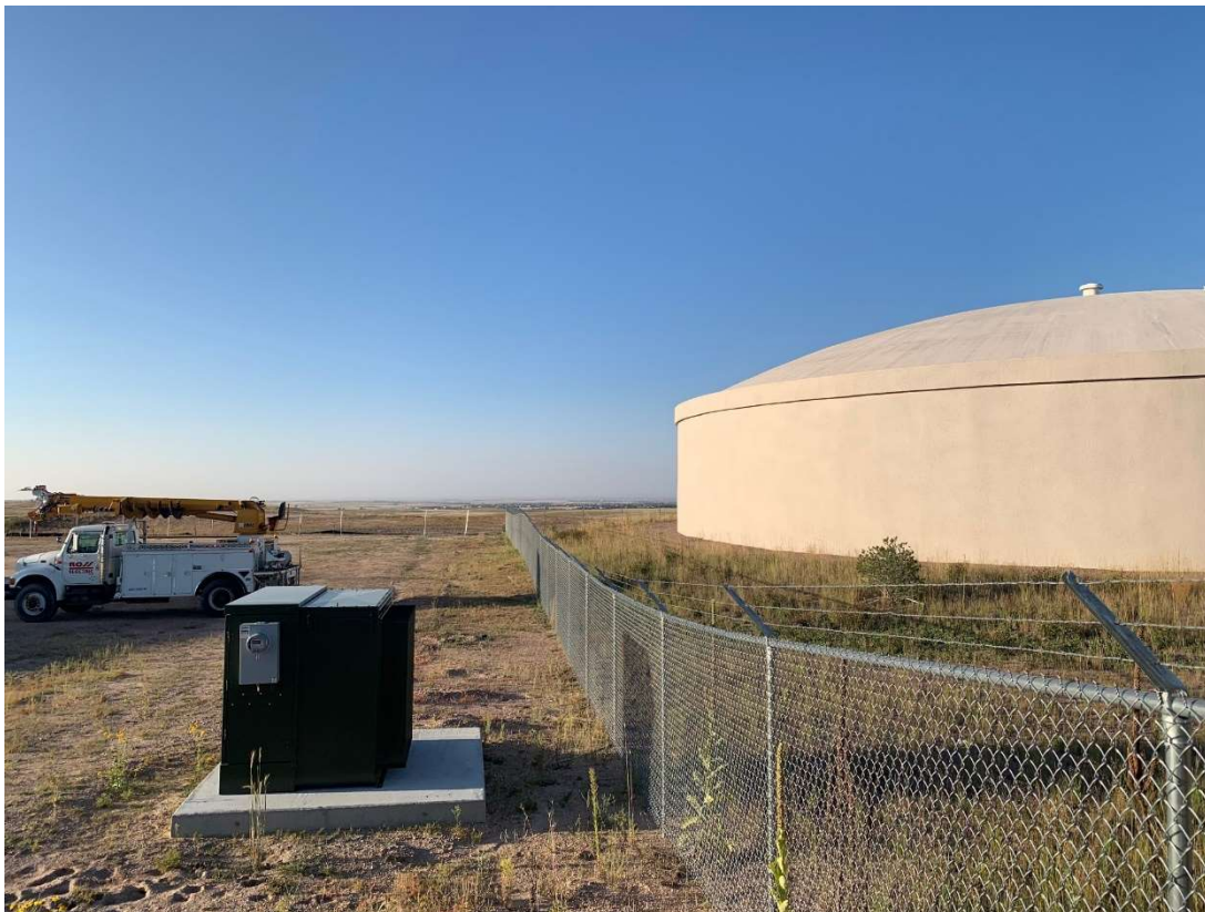
Picture taken 9/8/23 looking south on property line between tanks
