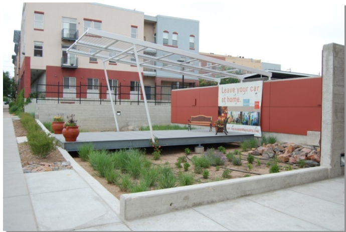
Photograph B-1. This recently constructed rain garden provides bioretention of pollutants, as well as an attractive amenity for a residential building. Treatment should improve as vegetation matures.
