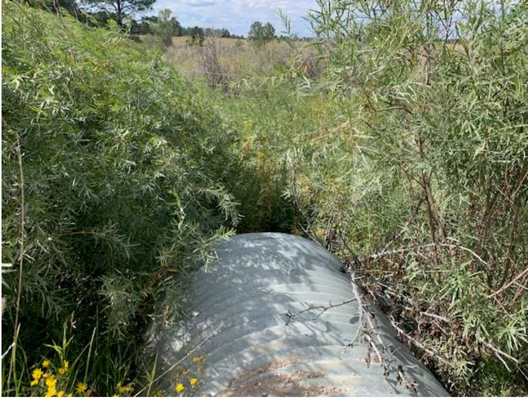
SAND CREEK REACH 9 - LOOKING UPSTREAM (EX. 60" CMP AT ARROYA LN.)
