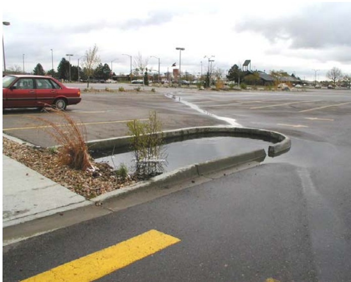
Photograph B-4. Runoff passed the upgradient rain garden, shown in Photo B-3, and flooded this downstream rain garden.
