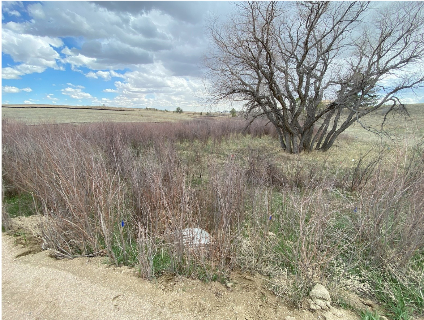
Final view from Arroya Lane looking into the willows in the floodplain with the culvert visible, facing south. There is no evidence of an OHWM present – no bed, no banks, no scour, no changes in sediment or topography – just a broad fluvial plain with willows.
