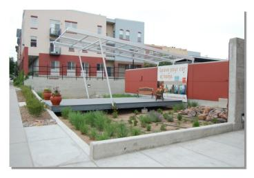
**Photograph B-1**. This recently constructed rain garden provides bioretention of pollutants, as well as an attractive amenity for a residential building. Treatment should improve as vegetation matures.
