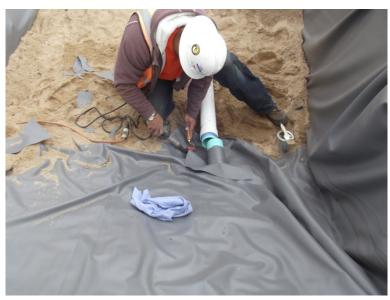
**Photograph B-3**. Ensure a water-tight connection where the underdrain penetrated the liner. The heat-welded "boot" shown here is an alternative to the clamped detail shown in Figure B-2.
