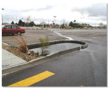
**Photograph B-4.** Runoff passed the upradient rain garden, shown in Photo B-3, and flooded this downstream rain garden.
