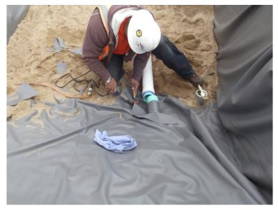
**Photograph B-3**. Ensure a water-tight connection where the underdrain penetrated the liner. The heat-welded "boot" shown here is an alternative to the clamped detail shown in Figure B-2.
