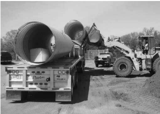
Lifting CMP off the flatbed with a front end loader and forks.
