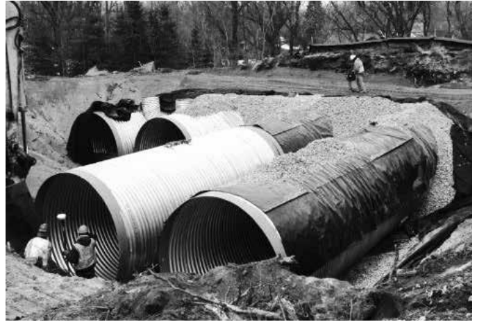
An HDPE liner is rolled out over the crown of the pipe prior to backfilling around the pipe.
