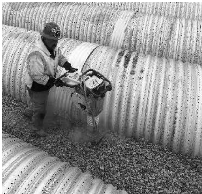
Compaction with vibratory equipment.
