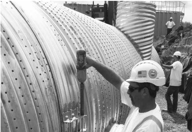
Tightening bolts on a corrugated band.
