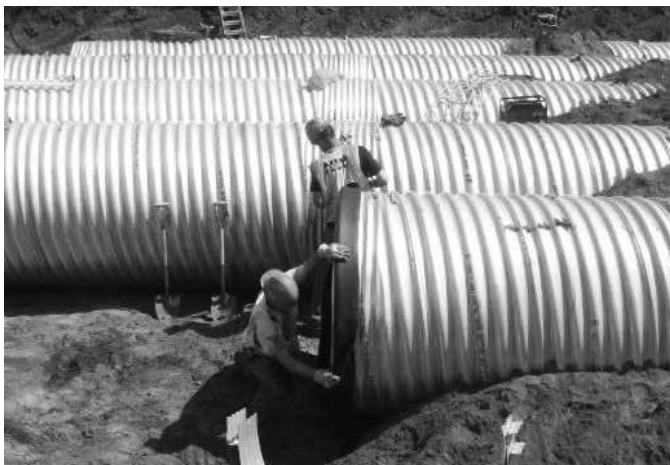
Installation of band with flat neoprene gasket.
