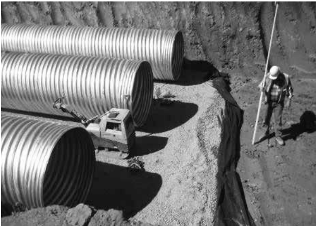
Site conditions may require 4" – 6" of imported granular material as pipe bedding.
