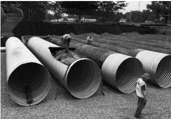
For large diameter pipes, the liner is shipped in rolls that are folded in half. The liner is rolled out over the crown of the pipe, unfolded, and covered over the pipe from the eight and four o'clock positions.
