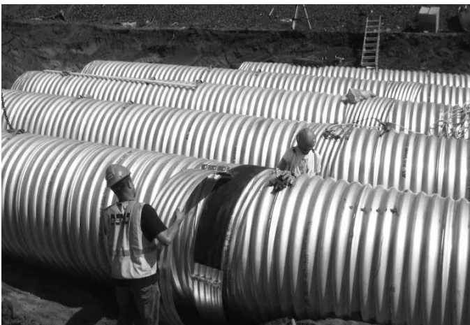
Tightening bolts on a corrugated band.
