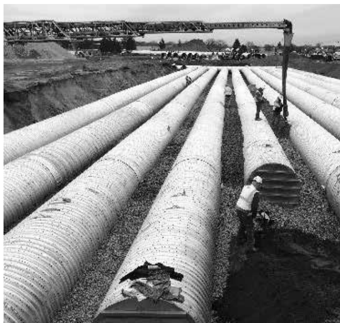
Placing backfill with a conveyor.
