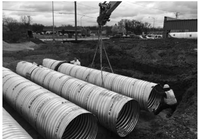
Lifting ALT2 CMP with nylon slings.
