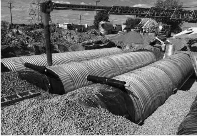
An HDPE liner is rolled out over the crown of the pipe prior to backfilling around the pipe.
