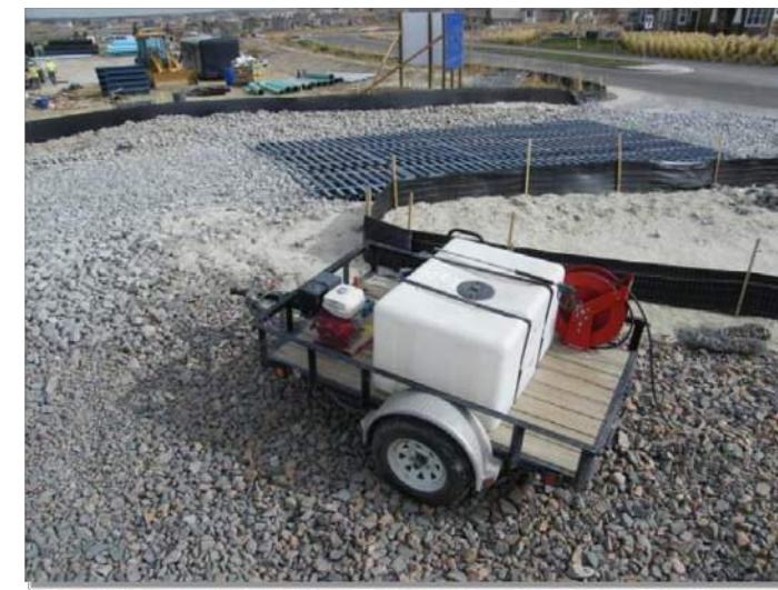
Photograph VTC-2. A vehicle tracking control pad with wheel wash facility. Photo courtesy of Tom Gore.
