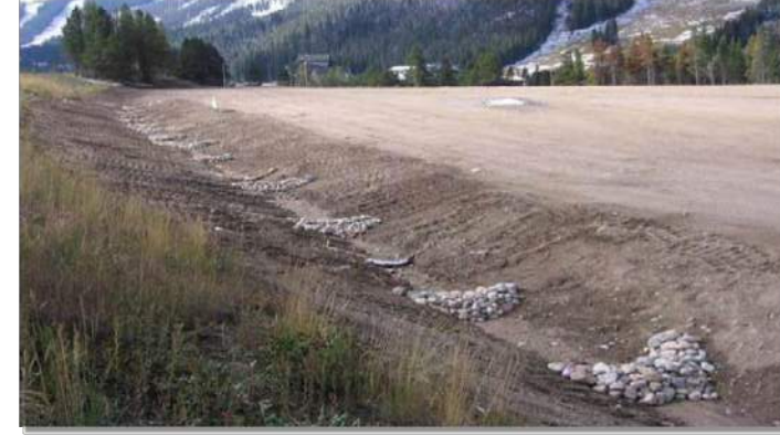
Photograph CD-1. Rock check dams in a roadside ditch. Photo courtesy of WVE.
