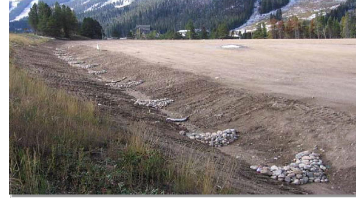
Photograph CD-1. Rock check dams in a roadside ditch. Photo courtesy of WVE.
