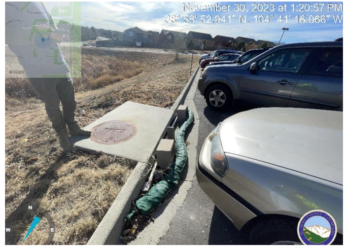
Photo 4: Inlet protection can be removed.
