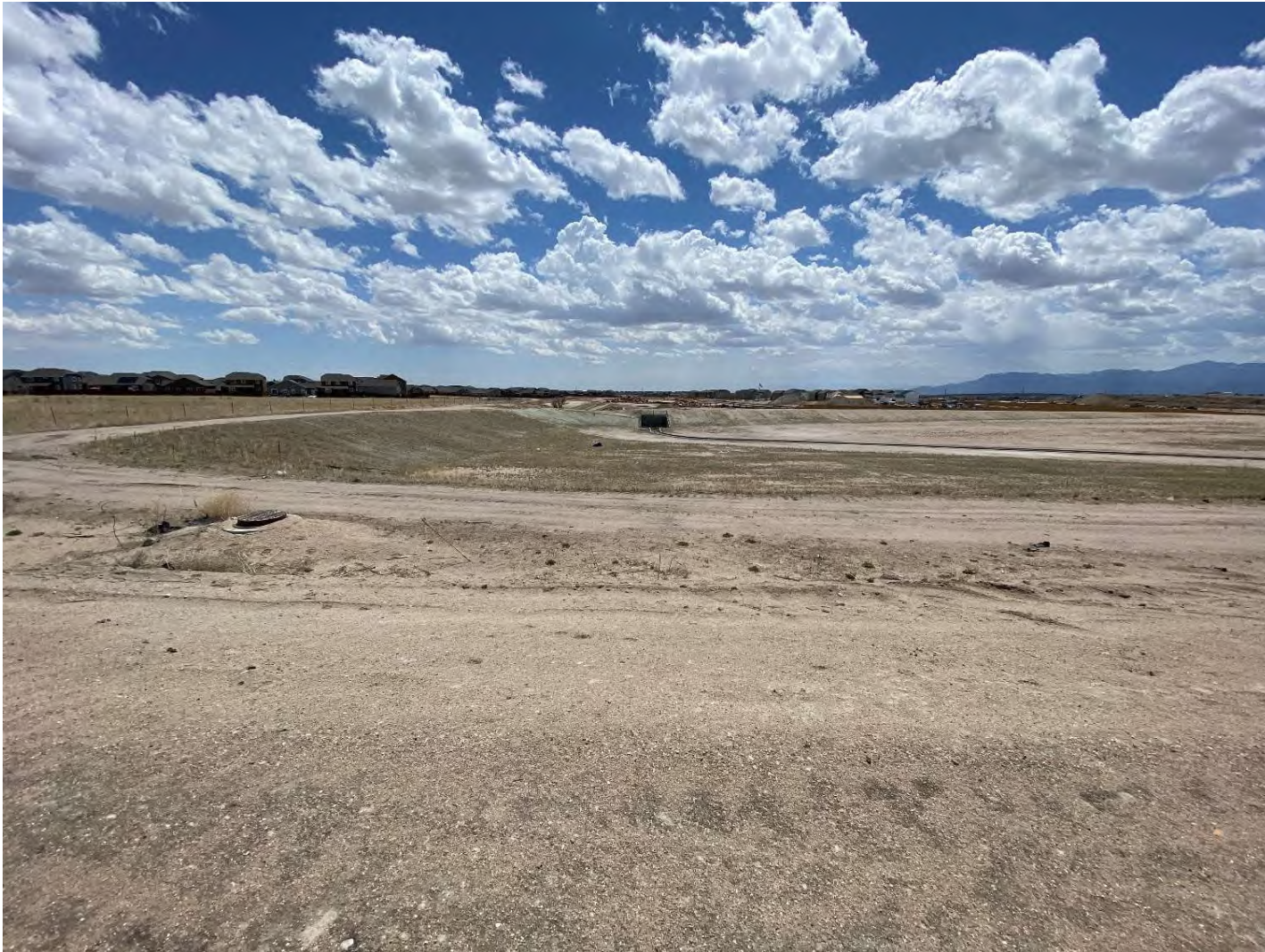
Extensive graded areas at the south end of the Project area, just north of the Aspen Meadows development; houses in this development can be seen from the righthand edge to the approximate center of the photo. The houses at left are from another offsite development.
