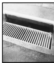
Directional 45-Degree Bar Grate
