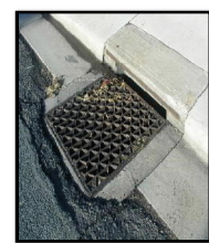
Reinforcing Riveted Grate
