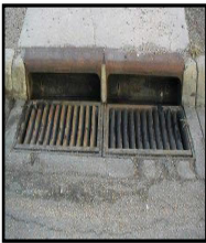
Bidirectional Cast Vane Grate
