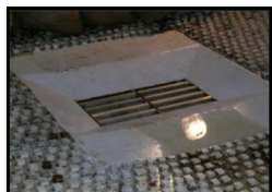
CDOT Type D Inlet Parallel (Flat & Depressed)
