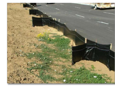
Photograph SF-2: When silt fence is not installed along the contour, a "hook" installation may be appropriate to force runoff to pond and evaporate or infiltrate in multiple areas rather than concentrate and cause erosive conditions parallel to the silt fence. Photo courtesy of Tom Coen.
