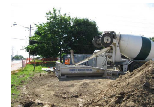
Photograph CWA-2. Prefabricated concrete washout. Photo courtesy of CDOT.
