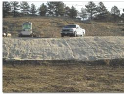
Photograph RECP-1. Erosion control blankets protecting the slope from erosion and providing favorable conditions for revegetation.
