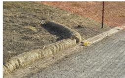
Photographs SCL-1 and SCL-2. Sediment control logs used as 1) a perimeter control around a soil stockpile; and, 2) as a "hook" perimeter control at the corner of a construction site.
