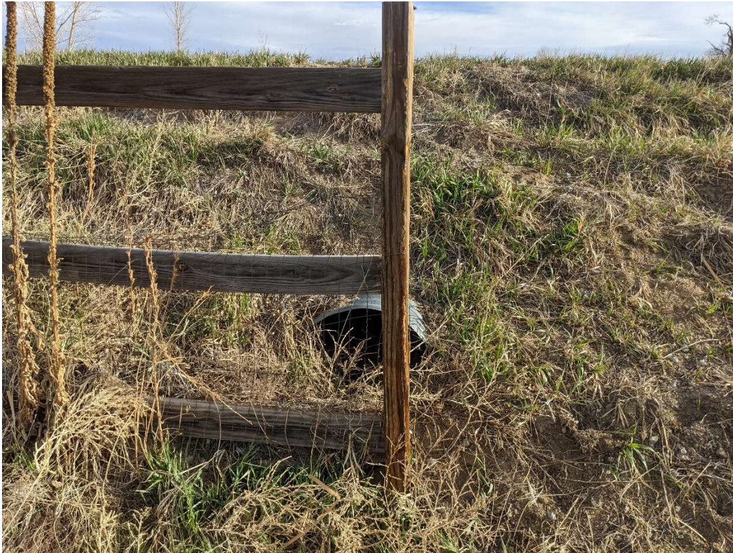
Figure 1: Storm Drain Culver Beneath Falcon Highway
