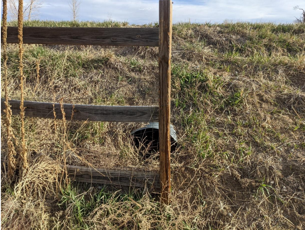
Figure 1: Storm Drain Culver Beneath Falcon Highway
