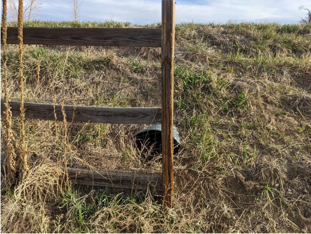
Figure 1: Storm Drain Culver Beneath Falcon Highway
