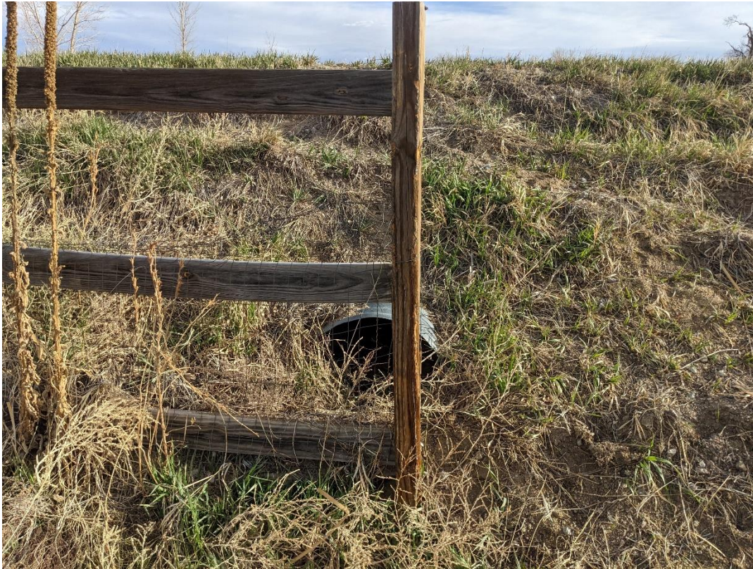
Figure 1: Storm Drain Culver Beneath Falcon Highway
