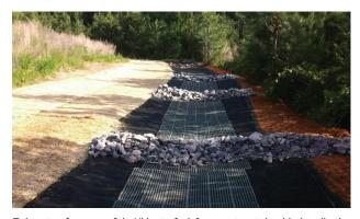
To boost performance of the VMax turf reinforcement mats in critical applications, combine with our ShoreMax<sup>®</sup> flexible transition mat to create a system that can dramatically elevate the permissible shear stress and velocity protection beyond many hard armor solutions.
